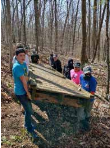
Installing a new bridge on the trail.
